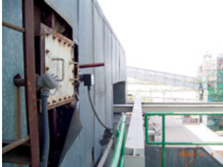
Accredited DynamicOpacity™ instrument monitoring Electro filters
