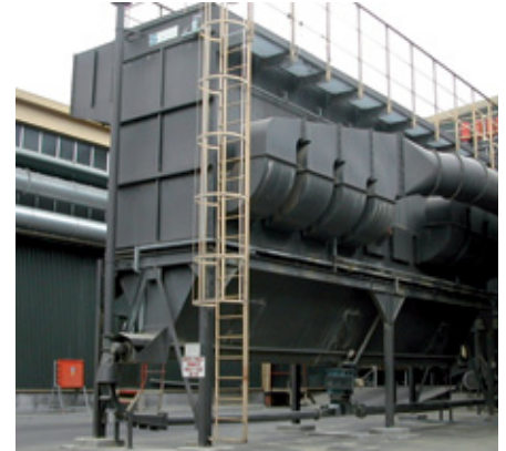
Filter chamber performance continuously monitored via a networked ElectroDynamic™ System
