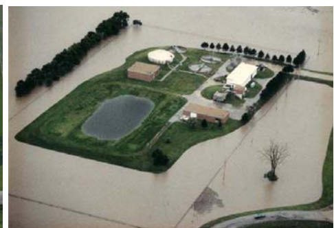
WWTP during flood conditions (photo taken prior to 1995 construction)
