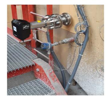
Material: Combustion gases: O<sub>2</sub> and CO
