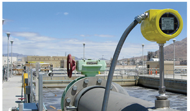
Figure 5: In outdoor, harsh desert sunlight, know the ambient conditions of your installation location
