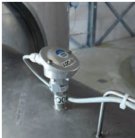
SIMPLE BROKEN BAG DETECTION
