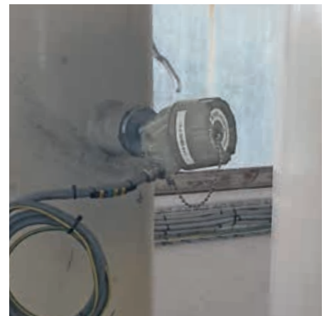
COMPACT SENSOR FOR BROKEN BAG DETECTION
