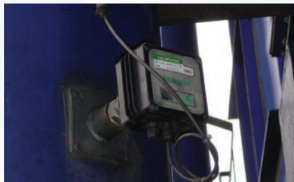
Carbon Black Filter Plant with Electrodynamic Sensors
