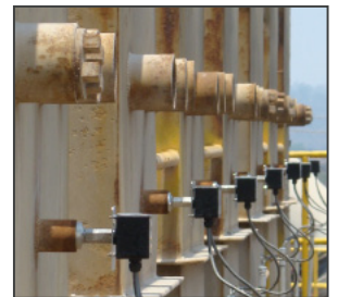
Individual filter chamber performance continuously monitored via a networked ElectroDynamic™ system
