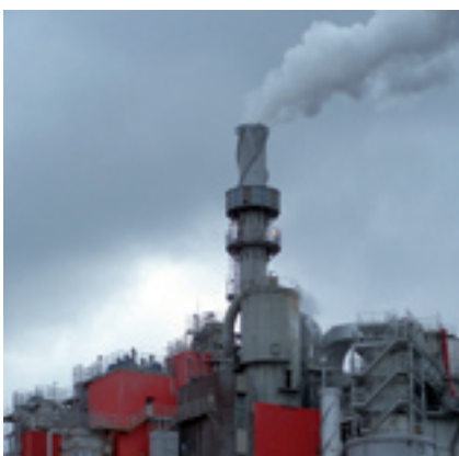
Electrodynamic monitoring of Detergent Manufacturing Plant
