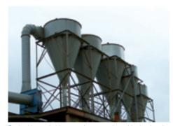
De-barking and chipper cyclones monitored by insulated Electrodynamic sensors
