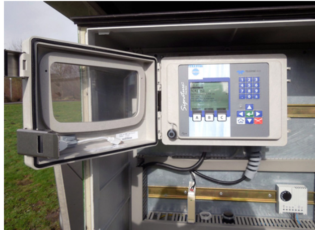
Stormwater pipe to be monitored & Signature Flow Meter
